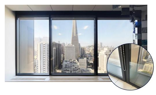
INOVUES SWR retrofit (buttjointed overlapmount) at One Maritime Plaza, San Francisco, maintains the daylight opening and does not interfere with the existing perimeter HVAC covers.
